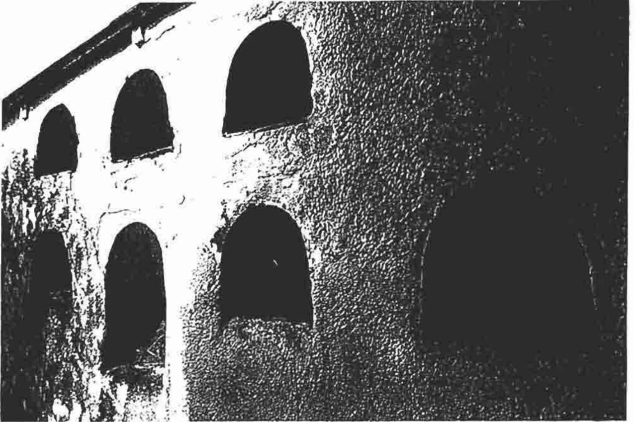
Fig. 2 Seven domed bores in barn end wall at North Tawton.
